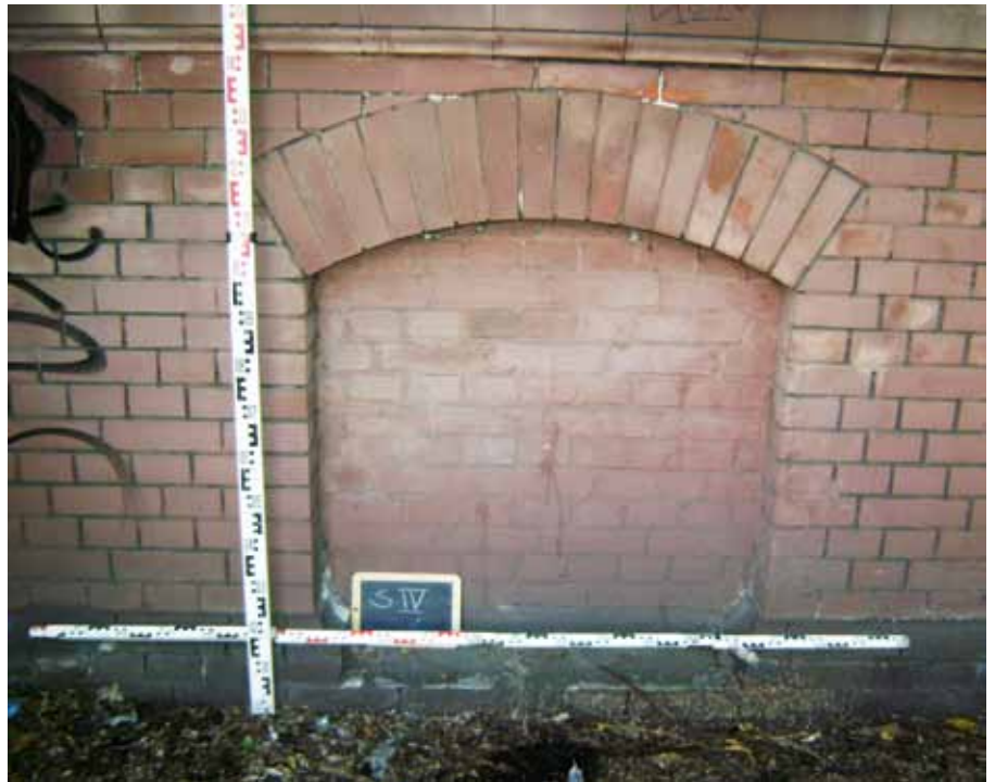
Fig. 7. Sealed cellar window SIV, possibly an attempt to convert the cellar into a makeshift air raid shelter.
