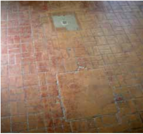
Fig. 6. The square base at the bottom of the picture was designed into the basket weave pattern as indicated by the change in pattern around the periphery of it. This differs from the later electrical construction at the top of the picture that worked around the brick pattern and filled the gaps with another material.
